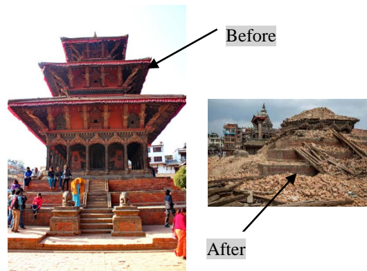
Figure 16. Harishankar temple before and after the earthquake.
