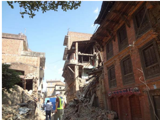
Figure 27. View of the spot in Fig. 15 after the earthquake.
