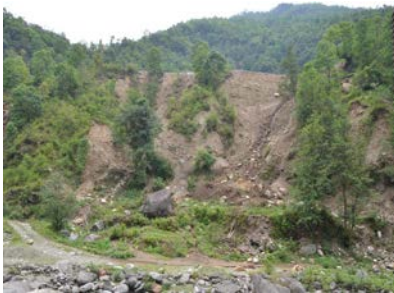
(b) Landslide in the right bank of Headworks
