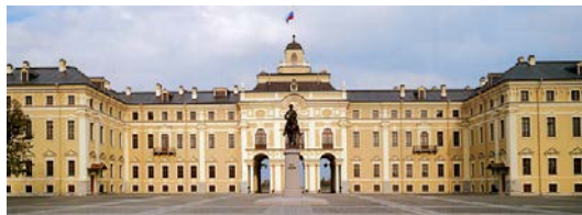
Figure 13. Konstantinovsky Palace, south facade. View after a final reconstruction stage (July 2003).
