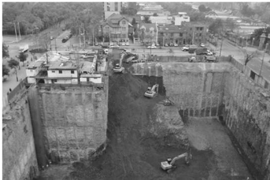
Figure 2. Deep excavation of 26,5m.
