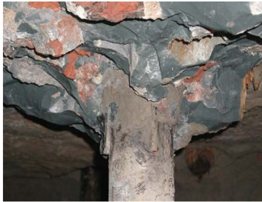
Figure 11. Bored pile with tube reinforcement viewed from underneath foundation.
