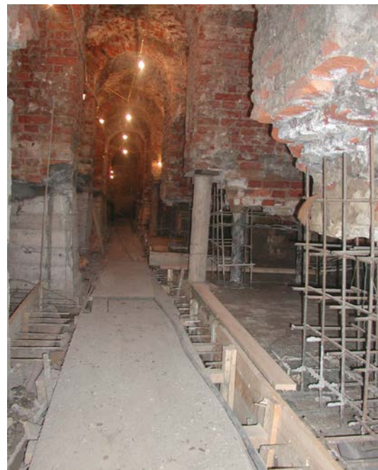
Figure 10. Deepening of the basements by 1.0-1.5 m.
