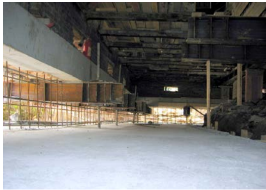
Figure 17. Construction of the top slab.
