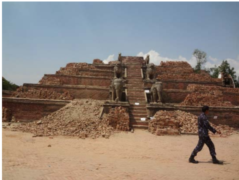
Figure 18. Vatsala Durga temple after the earthquake.
