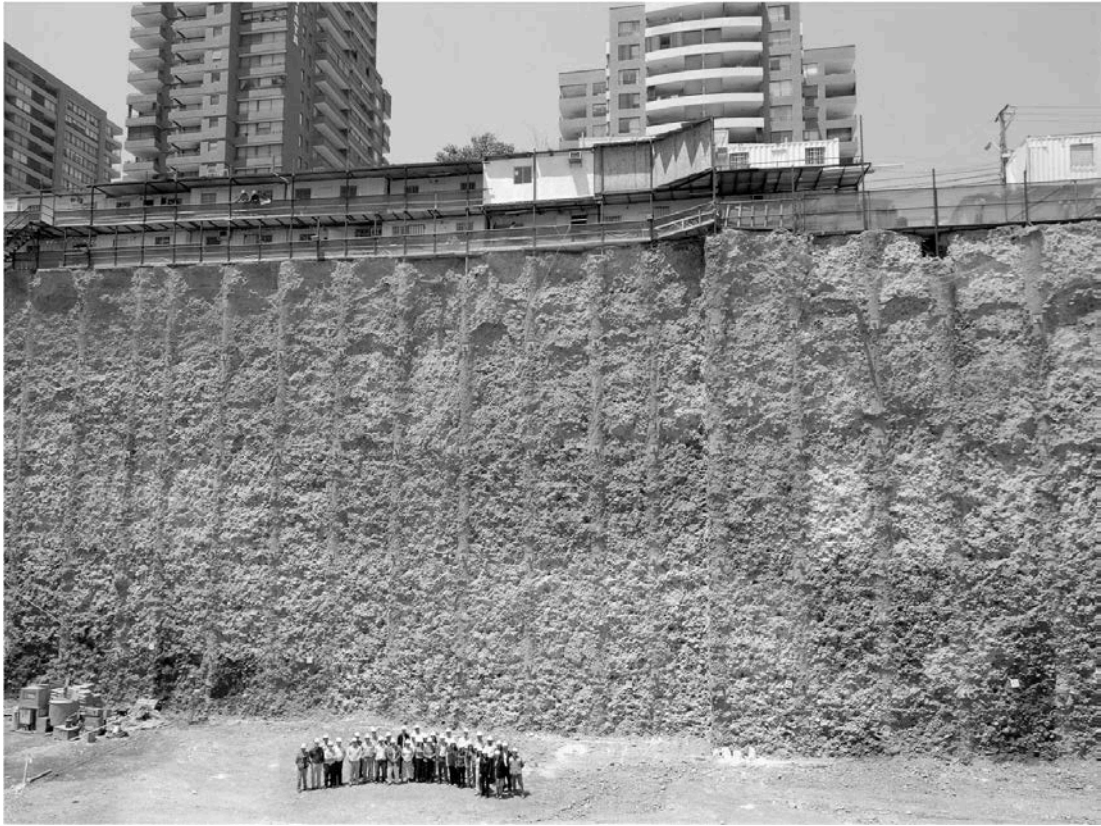
Figure 11. Deep excavation of 28 meters.
