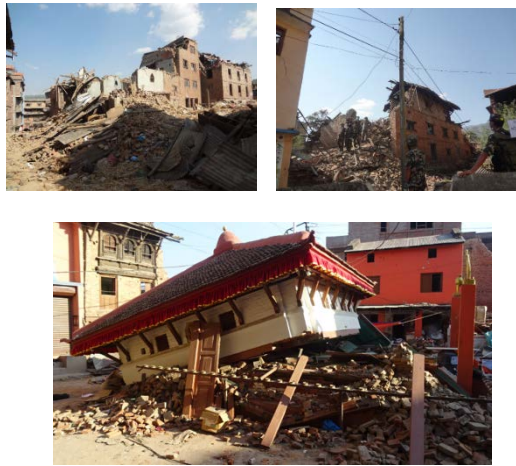
Figure 28. Few selected collapsed structures in the town.
