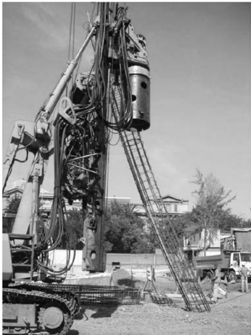
Figure 4. Installation of the pile reinforcement cage with the inclinometer tube attached
