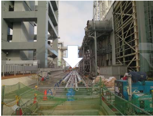
Fig. 6 Pipes for ground freezing around nuclear reactor building
