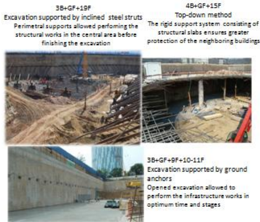
Figure 2. Examples of deep excavations designed by Popp & Asociatii Inginerie Geotehnica
