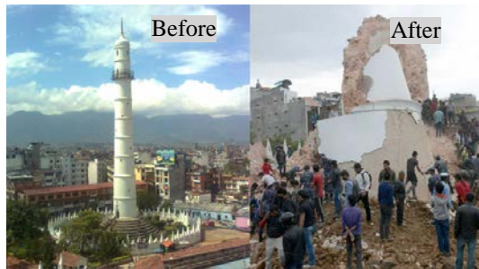
Figure 14. State of damage of Dharahara tower.
