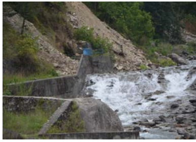
(a) Landslide in the upstream of intake
