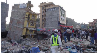
Figure 29. A typical case of damage to comparatively short buildings.
