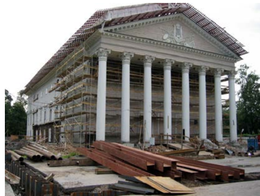
Figure 14. Kamennooostrovsky Theatre during reconstruction.
