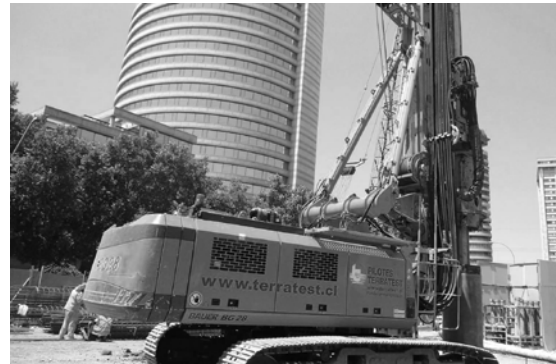
Figure 3. Bored cased piles being executed
