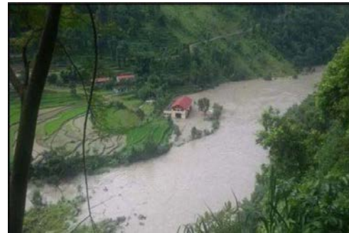
Figure 33. Submerged power station (Courtesy: Sanima Hydropower Ltd., Kathmandu)
