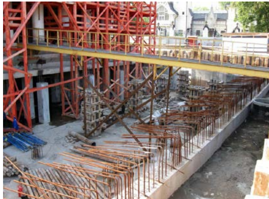
Figure 20. Constructing the underground structure.
