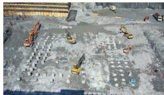
Figure 11. Trimming of PRD pile head
