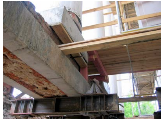
Figure 16. All loads have been redistributed. Old foundations removed.
