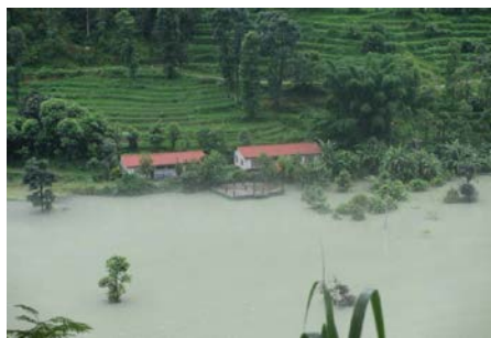
(b) After the landslide
