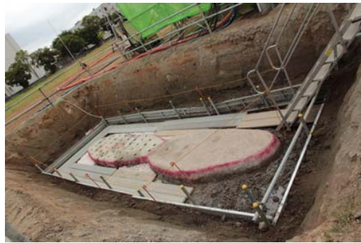
Fig. 5 Excavated trial underground wall
