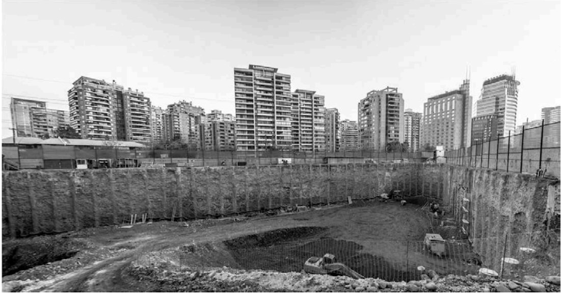
Figure 13. Parque Oriente building excavation completed.
