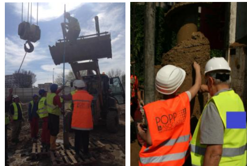
Figure 6. Images from work sites assisting for encountered conditions
