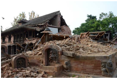
Figure 23. One of the collapsed temples in Changu Narayan.
