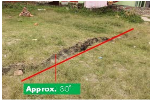
(a) Observed ground fissuring
