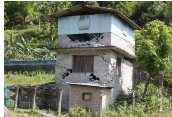
(c) Operator's camp at headworks
