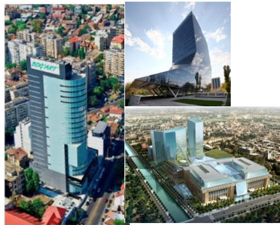
Figure 1. Photographs of representative buildings designed by Popp & Asociatii
