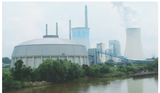
Figure 1. New circular coal storage at power station.
