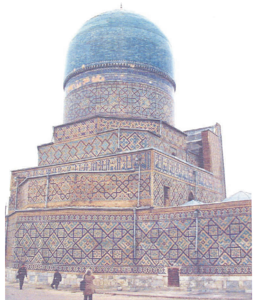
Fig. 1. Western wall of Tilla-Kori mosque.
