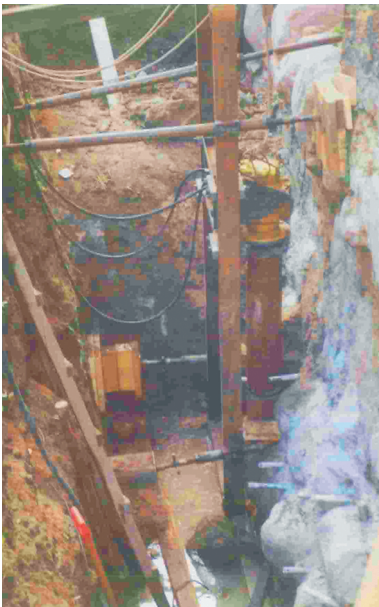
Figure 9. Simple screw driving equipment for drilled spiral piles.
