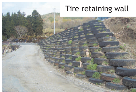
Figure 1. Tire retaining wall in Okirai
